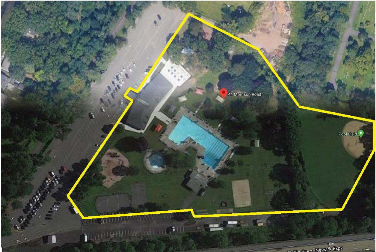
The Pool Facilities consist of the grounds and facilities outlined above.
